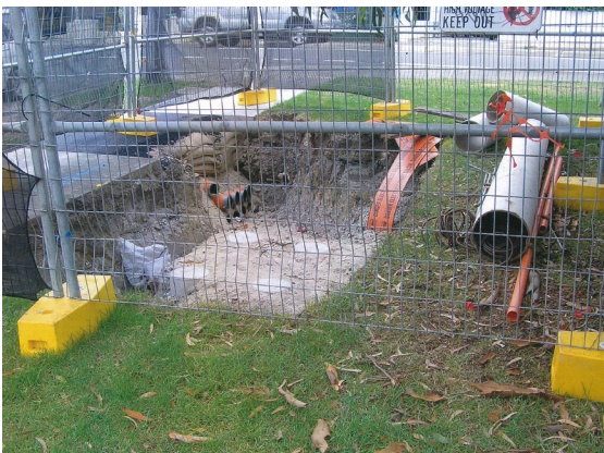
Figure 8 - An open excavation with barricades
