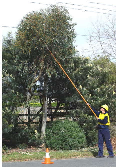
Figure 123 - CAVC work from groundline position ensuring insulated tool does not extend beyond the height of overhead high voltage powerlines.
