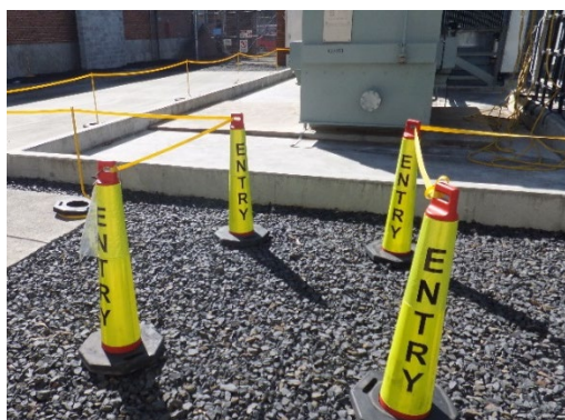
Figure 79 – A photograph and diagram illustrating correct entry to a safe work area with the entrance corridor tape formed at right angles to the safe work area.
