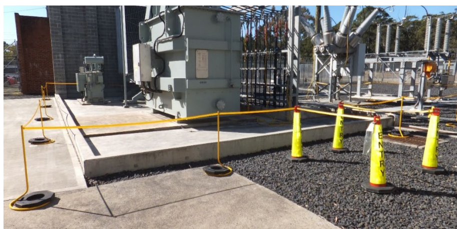
Figure 81 – A typical application of barrier-in method
