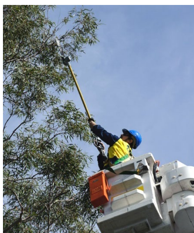
Figure 70 – A vegetation control worker a HV insulated hydraulic cutting saw
