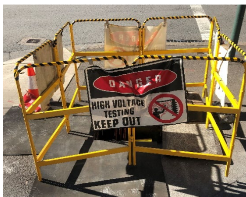
Figure 128 – Pedestrian barrier with black and yellow rail and danger notice
