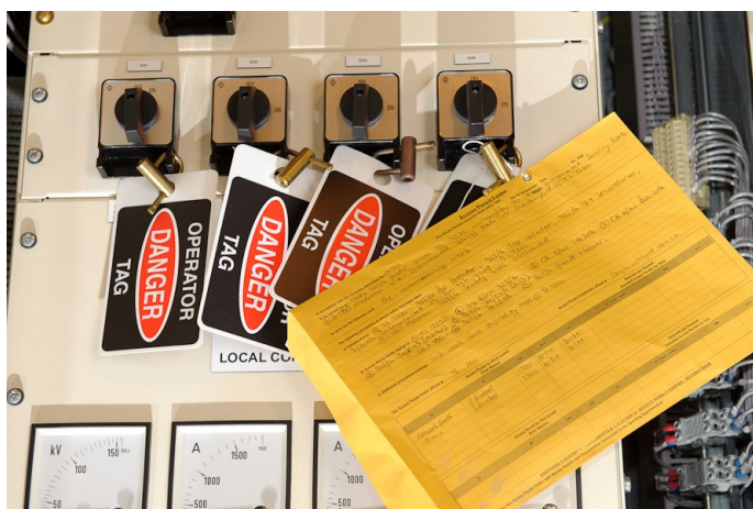
Figure 6 - Access permit folder at a worksite
