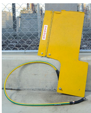
Figure 63 – An earthed screen for Hazemeyer switchgear
