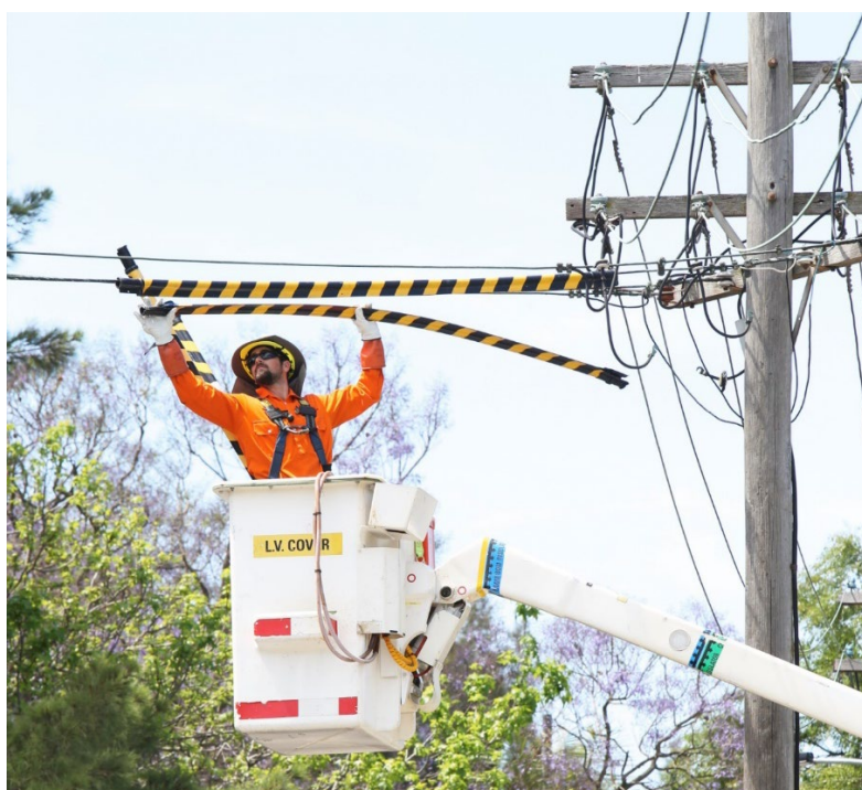
Figure 102 – Applying temporary insulation to low voltage overhead mains
