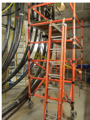
Figure 77 - Using lightweight fibreglass scaffolding
