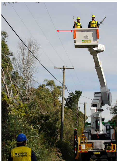
Figure 122 - CAVC workers allowing for minimum approach distances using an observer.
