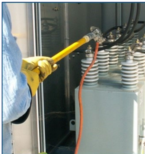
FIGURE 6: WAIT 15 MINS TO DISCHARGE BEFORE APPLYING EARTHS
