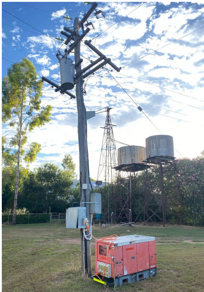
FIGURE 7: LEGACY SITE WITH CUSTOMER ASSETS ATTACHED TO ESSENTIAL ENERGY ASSETS
