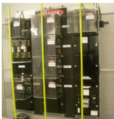
Figure 30 - A screen over exposed LV apparatus in a substation.
