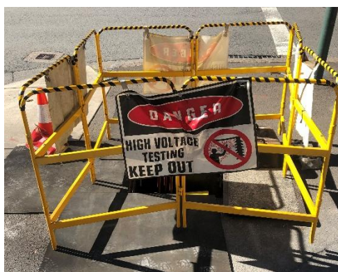
Figure 92 – Pedestrian barrier with black and yellow rail and danger notice
