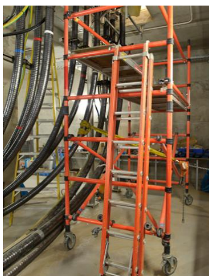
Figure 44 – Non-conductive (fibreglass) scaffolding in a substation
