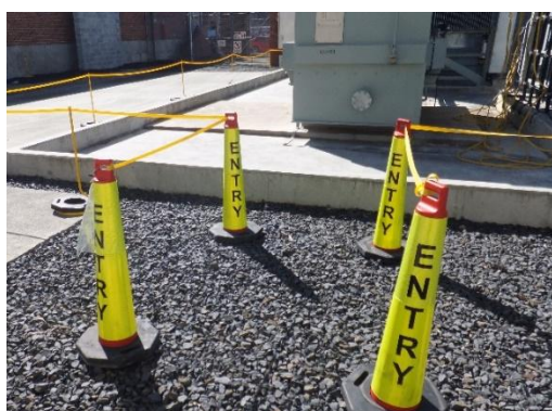
Figure 46 – A photograph and diagram illustrating correct entry to a safe work area with the entrance corridor tape formed at right angles to the safe work area.
