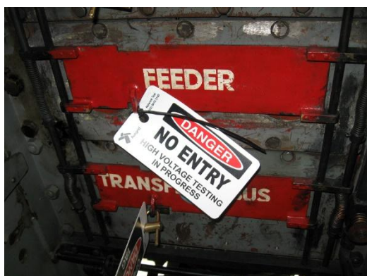
Figure 91 – HV testing tag applied
