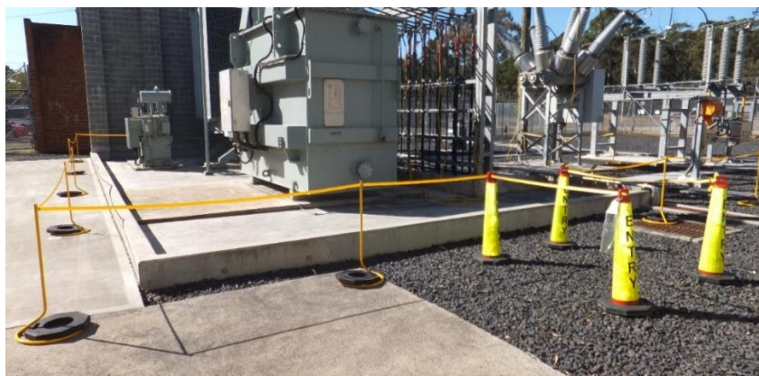
Figure 47 – A typical application of barrier-in method in an outdoor switchyard
