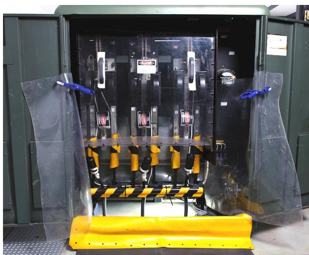
Figure 33 - LV temporary insulating covers and an insulating mat at a kiosk substation
