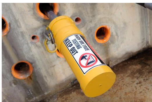
Figure 89 - Lockable cable termination with danger notice
