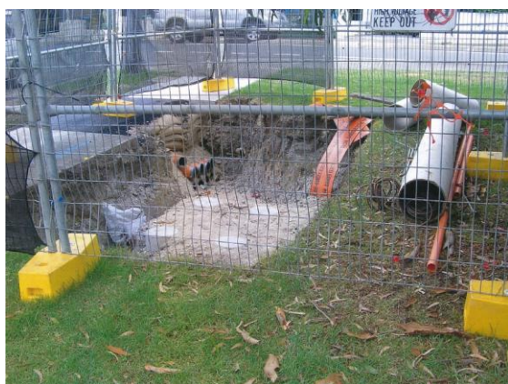
Figure 83 - An open excavation with barricades
