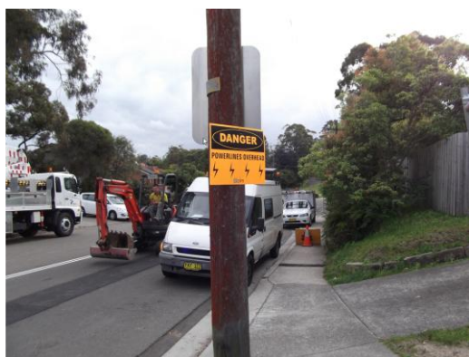
Figure 61 - Temporary 'Powerlines Overhead' warning sign
