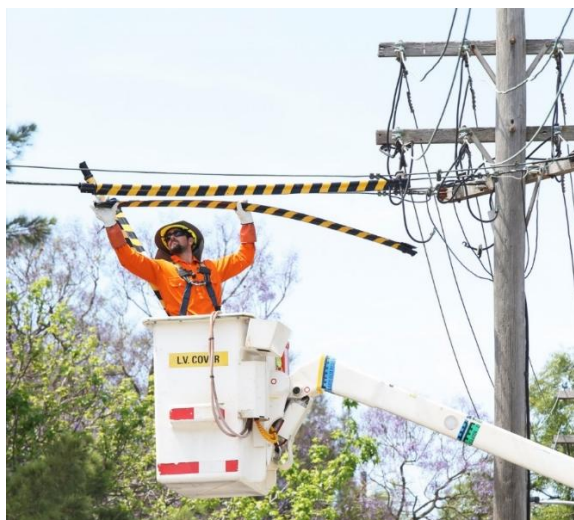
Figure 71 – Applying temporary insulating covers to low voltage overhead mains
