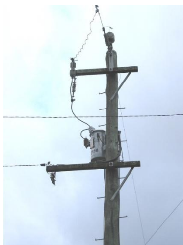
Figure 80 – A SWER substation
