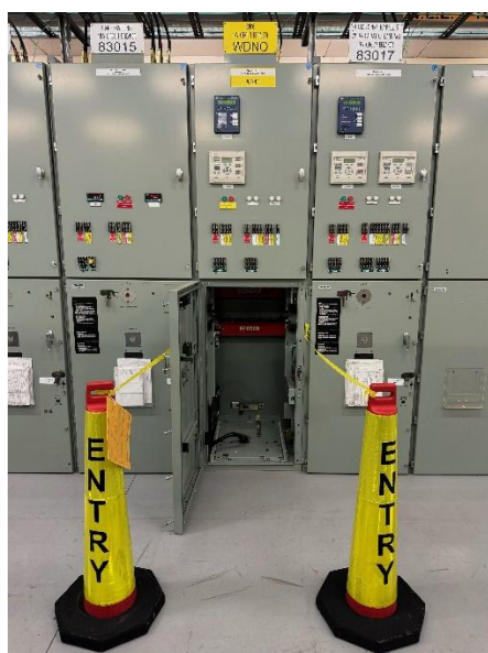
Figure 48 – An example of a barrier-in method used on indoor metal-clad switchgear
