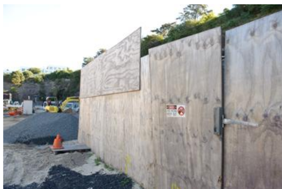
Figure 42 – An example of hoarding used to prevent workers encroaching MSWD
