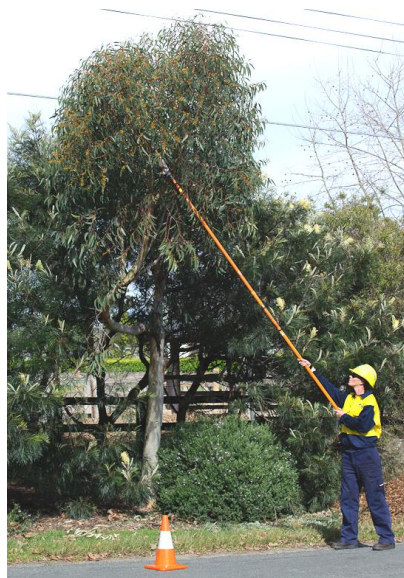
Figure 87 - CAVC work from groundline position ensuring insulated tool does not extend beyond the height of overhead high voltage powerlines.
