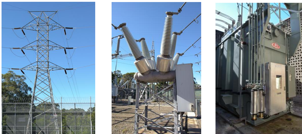
Figure 64 - Various parts of the network used by Ausgrid to supply electricity — overhead lines, a circuit breaker, and a transformer.
