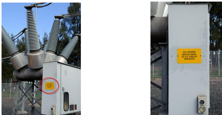
Figure 52 - Labelling on typical mains and apparatus
