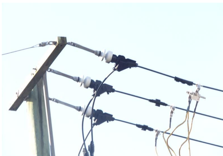
Figure 81 – HV covered conductors with earthing and short-circuiting equipment installed
