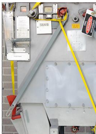
Figure 97 - Interlock engaged to prevent access to cable end box.
