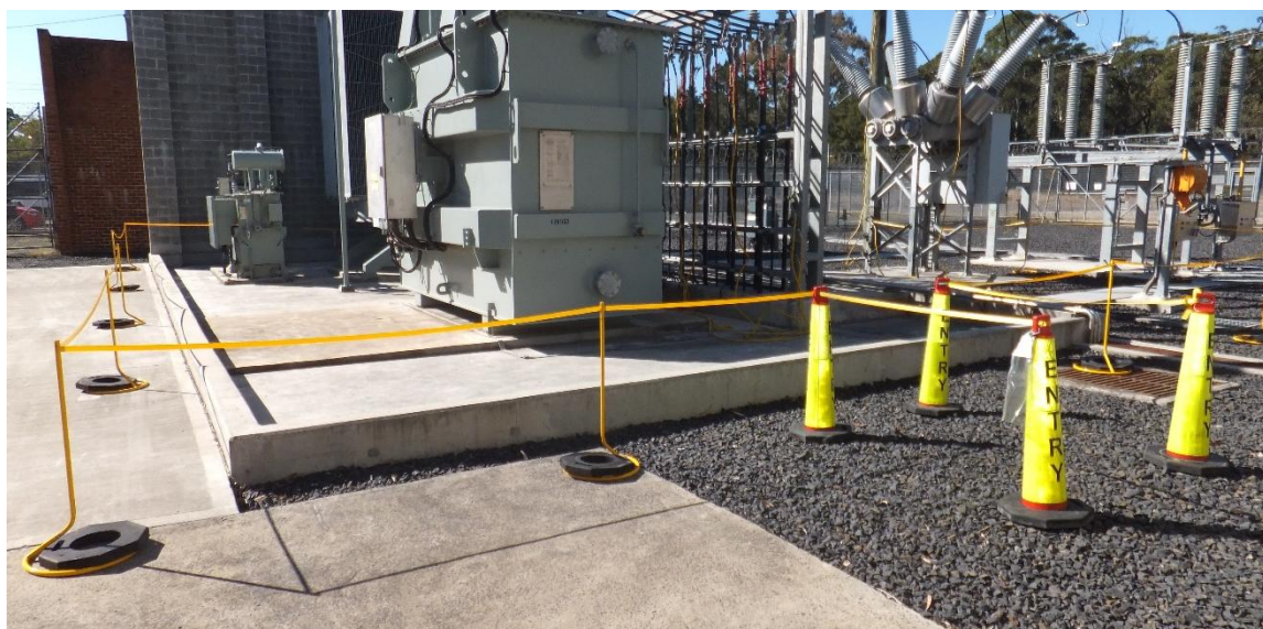
Figure 45 – An example of a safe work area defined by a yellow tape barrier (barrier-in method).
