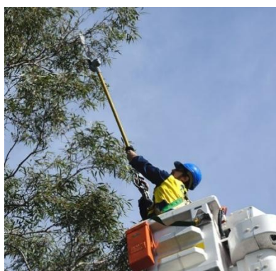
Figure 38 – A vegetation control worker a HV insulated hydraulic cutting saw
