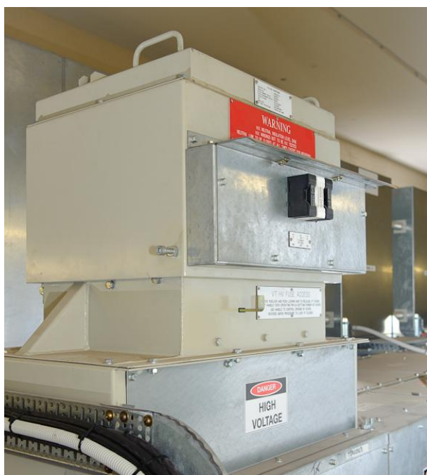
Figure 96 - 11kV—110V voltage transformer
