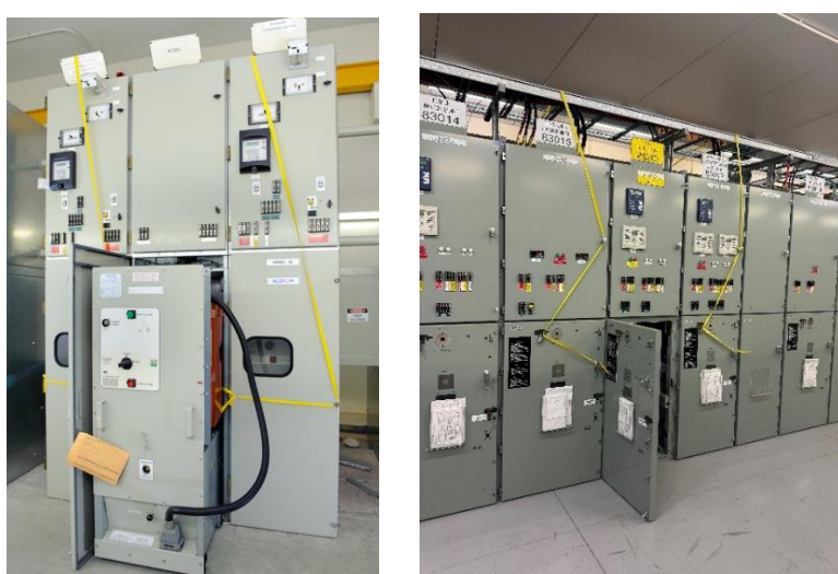
Figure 50 – Examples of barrier-out method used on indoor metal-clad switchgear
