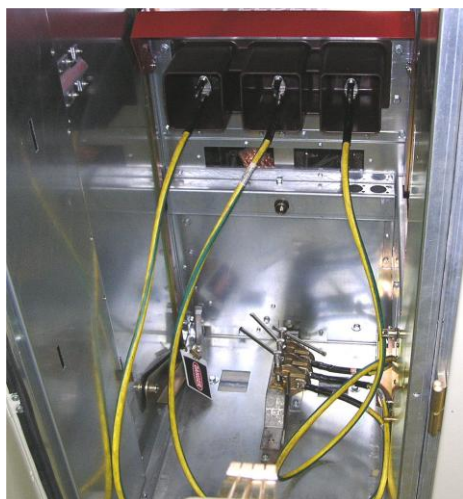
Figure 78 – Earthing applied to 11kV horizontal racking switchgear
