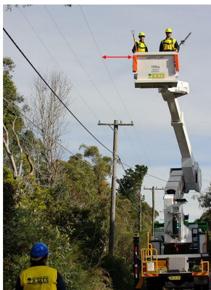
Figure 86 - CAVC workers allowing for minimum approach distances using an observer.
