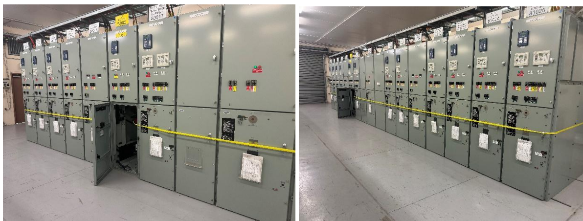
Figure 49 - An example of barrier-out method used on indoor metal-clad switchgear.
