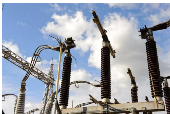
Figure 72 – Open 132kV isolator with closed earthing switch
