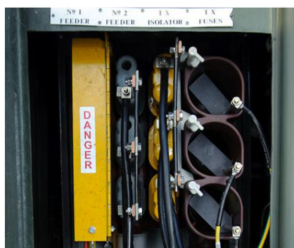
Figure 32 – An earthed screen in place covering live feeder spouts (note the busbar is earthed)
